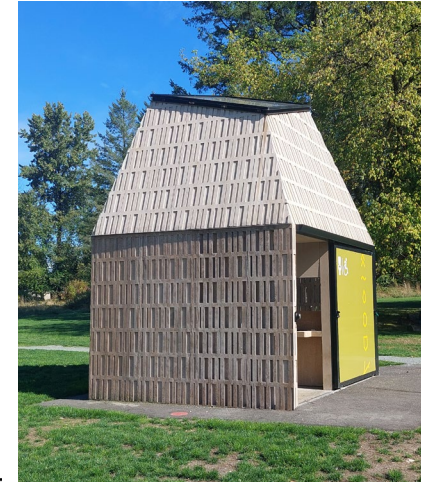
Image of washroom facility at Forsyth Park
